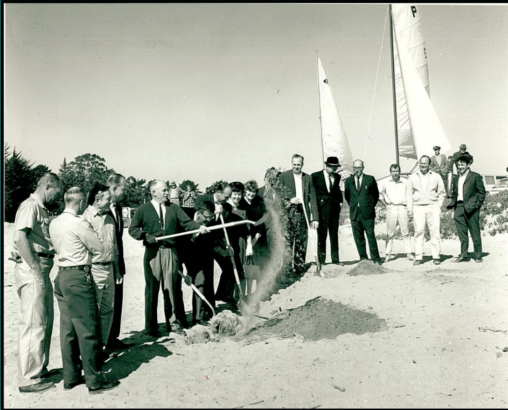
Groundbreaking for O'Neill Building, 1965
